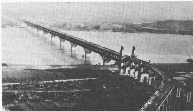
The Nanking Yangtze River Bridge
