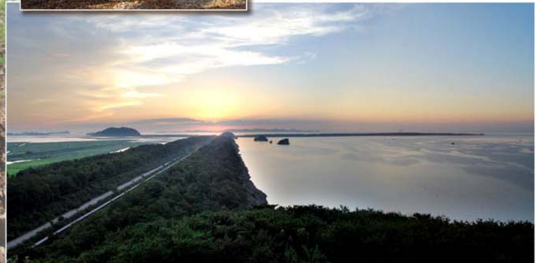
Muck is removed by the long-distance conveyor belt
