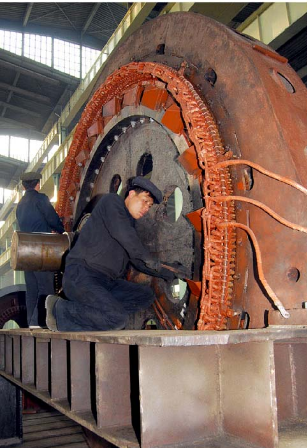
Assembling of an electric motor.
