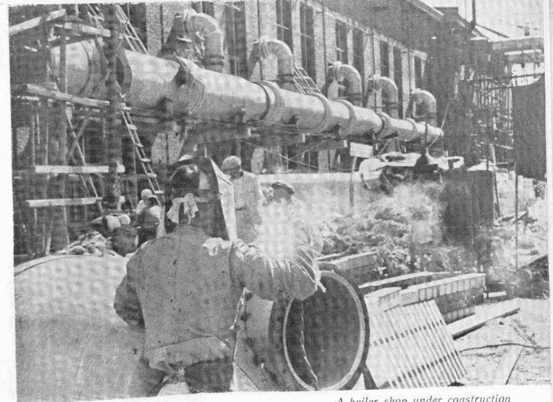
A boiler shop under construction
