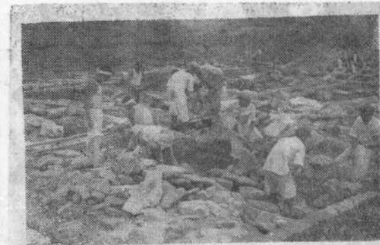
Groundwork for miners' apartment
