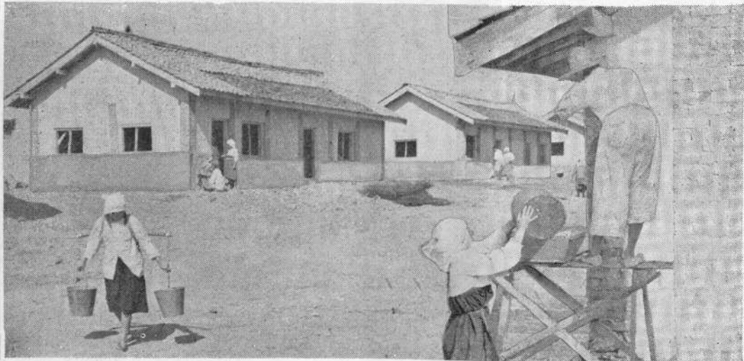
Finishing touch is being given to new dwelling houses
