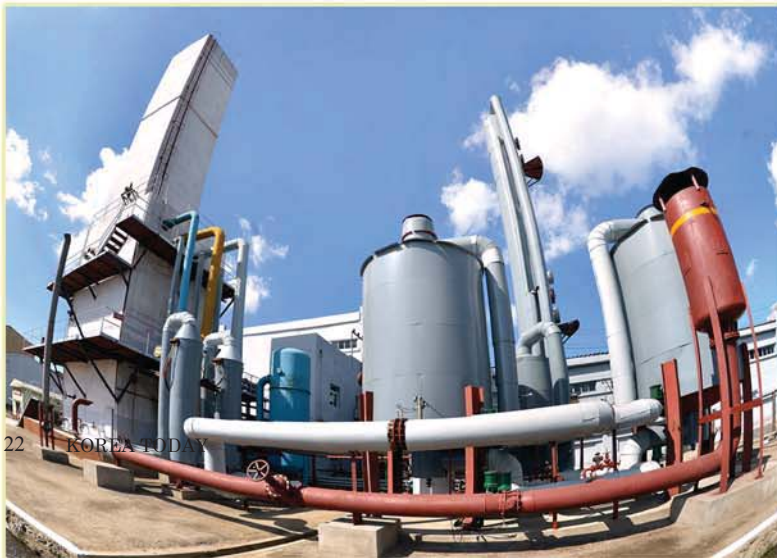
A view of oxygen plant workshop No. 1.
