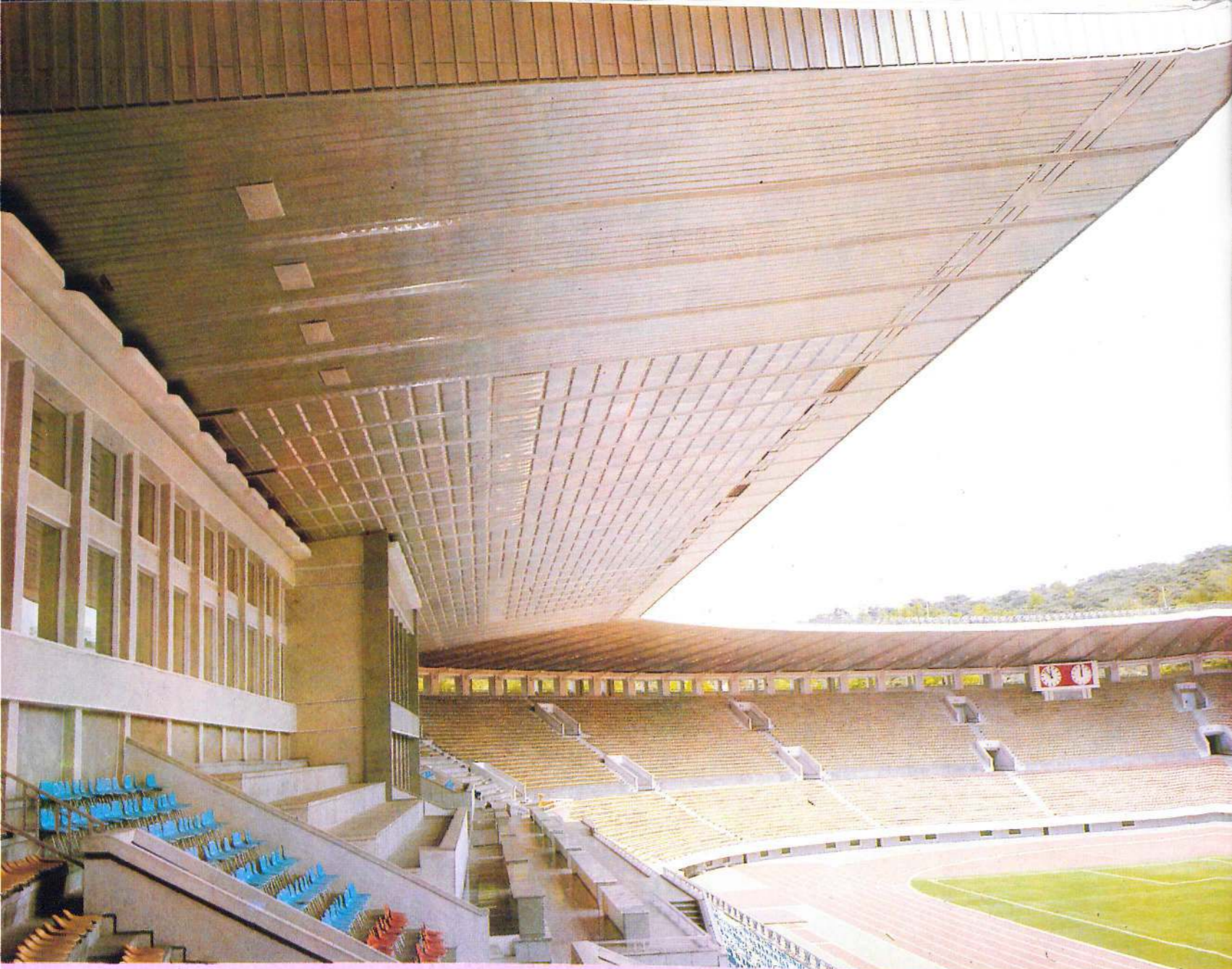
The grandstand with pent roof
