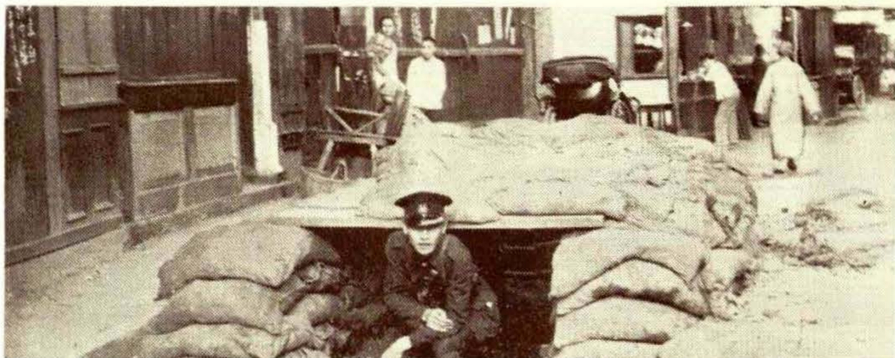
One of the smaller shelters, completed, with a member of the Police Bureau at the entrance. Charts showing how to use the shelters were posted prominently in Nantao.
