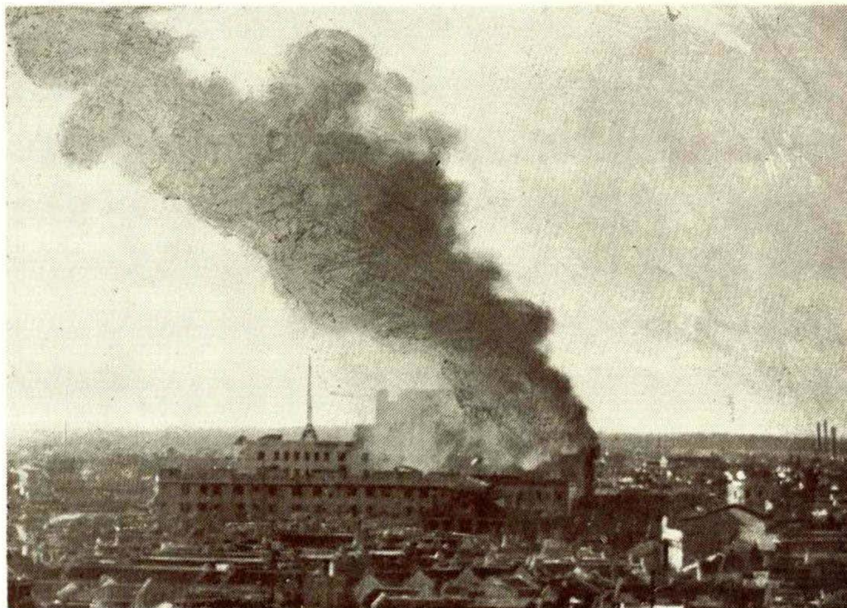
Destined to go the way of many other fine buildings in the war zone, the Administration Building was struck many times by shells on October 19. Finally, two incendiary bombs, dropped by a Japanese bomber set the east wing of the building afire, the flames spreading two storeys beneath. All day various types of Japanese aircraft, including new double-engined bombers, rained missiles on that area, until their objective was hit. This fire was the prelude to its downfall, which was accomplished a few days later.
