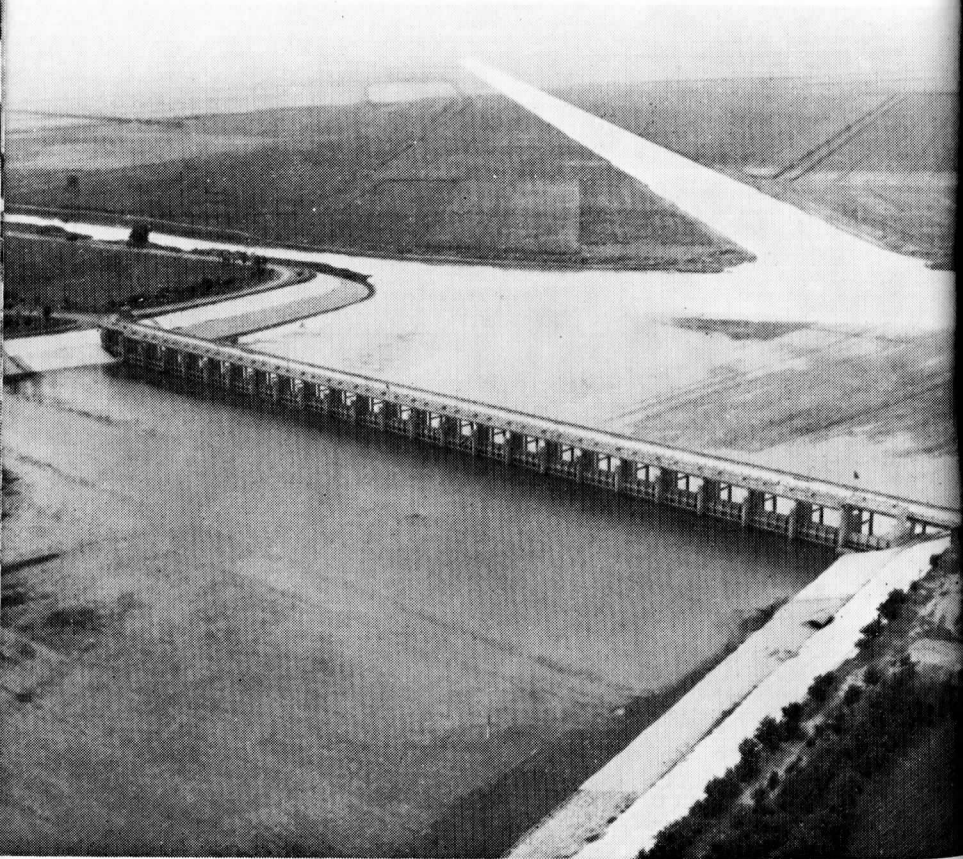
Headgate on the Tuliu Diversion Canal.
