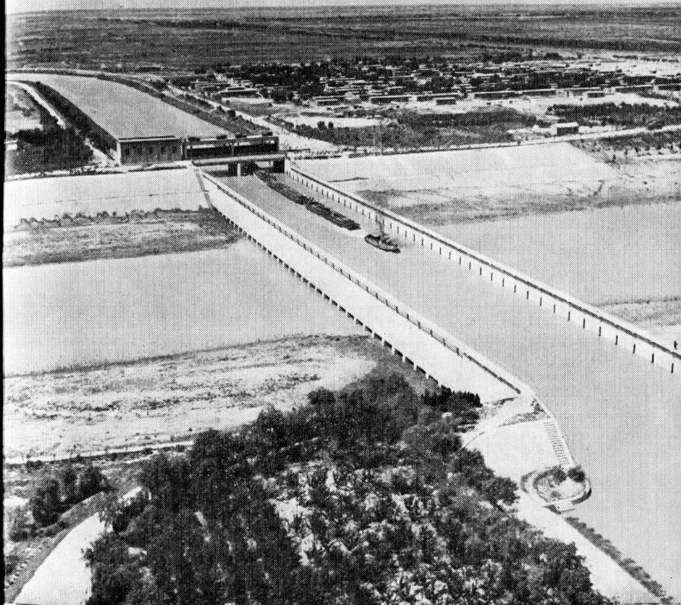
The New Tzuya main project across South Canal.
