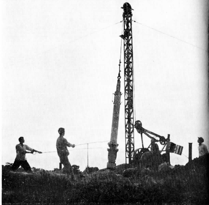
Working at the well-drilling site day and night.
