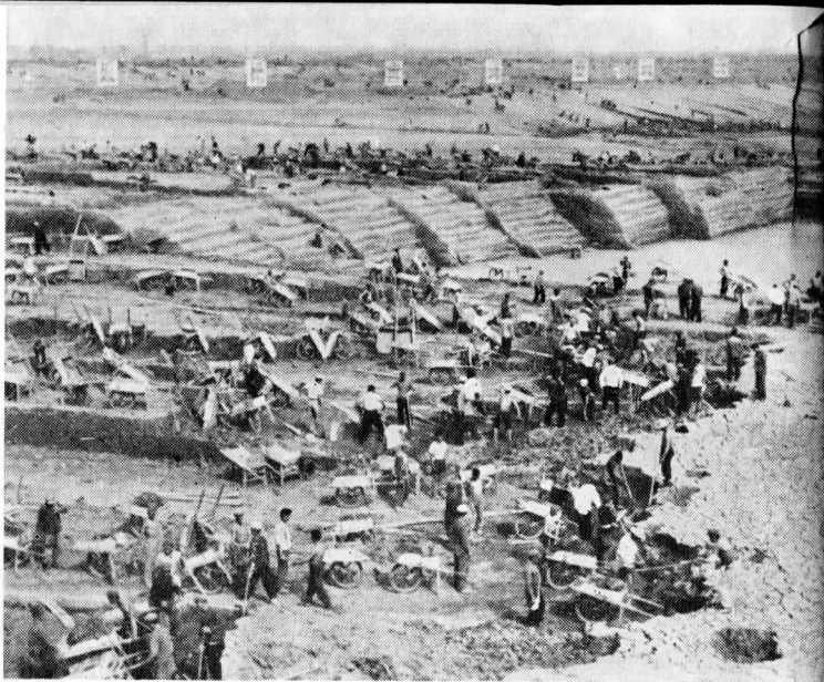
Dredging silt ( upper ).
