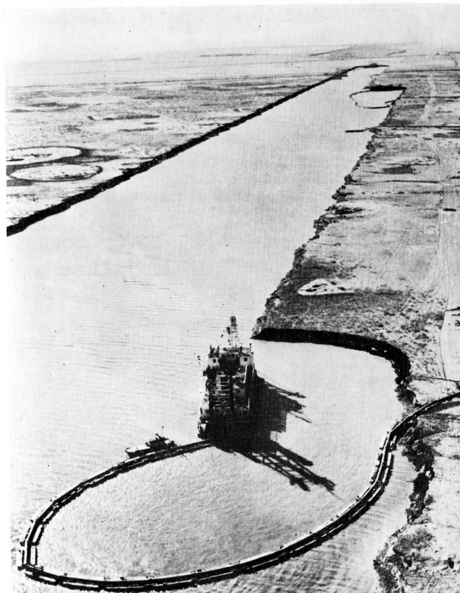
Dredger at work opening a new outlet to the sea.
