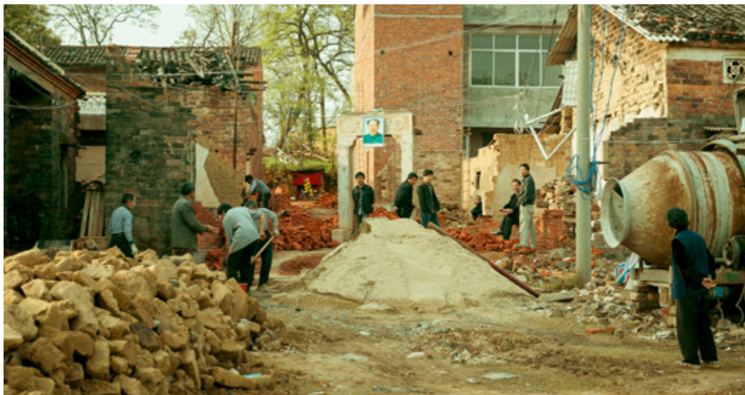
Construction work in a rural village in Hubei. PC: Tauno Tohk
