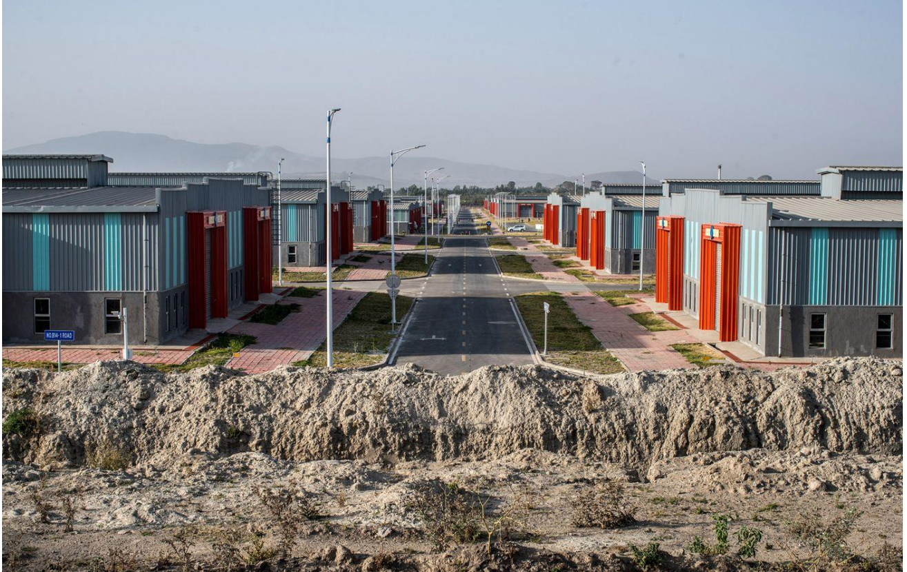
The facility, built on farmland, is the largest of four new textile and apparel centers. PHOTOGRAPHER: NICHOLE SOBECKI FOR BLOOMBERG BUSINESSWEEK
