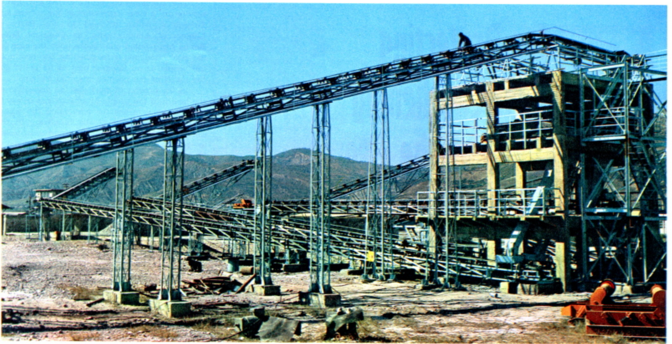
Work has begun on setting up the complex of buildings.
