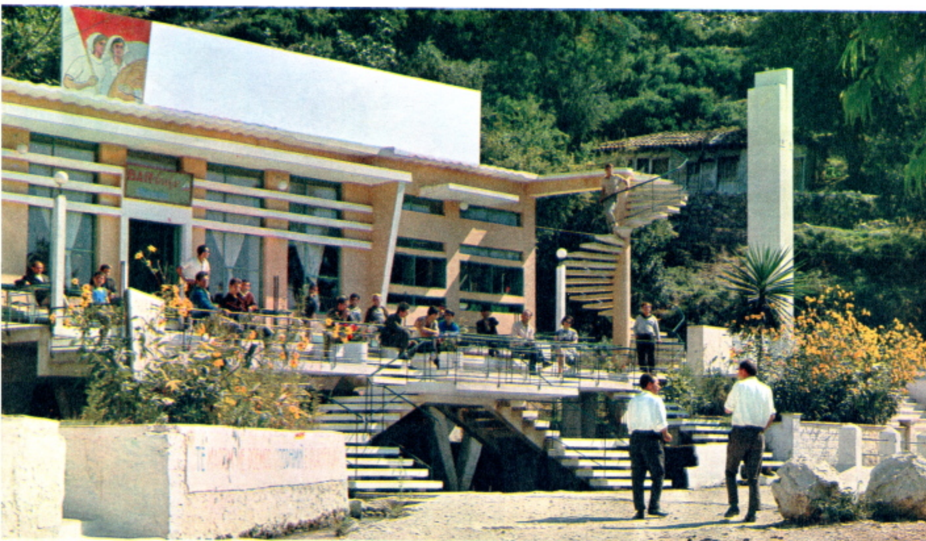
This new club house is built in the village of Borsh in Southern Albania.
