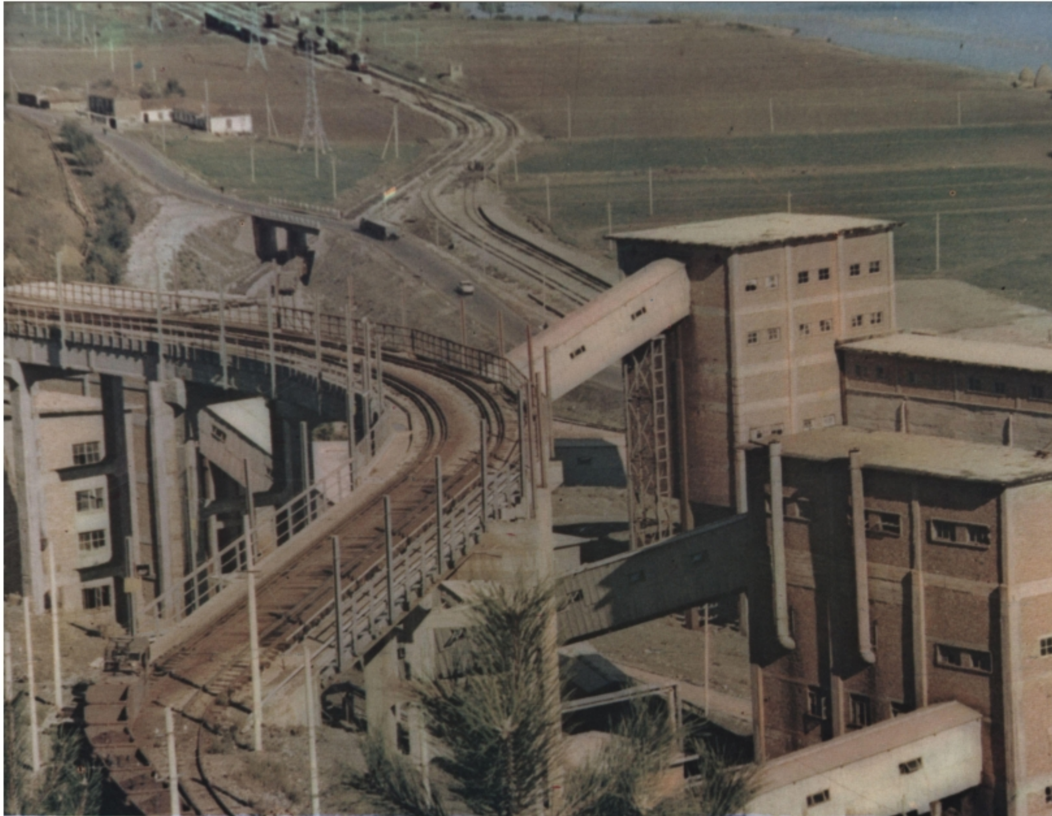
Fabrka e pasurimit të hekur-nikelit, Guri I Kuq, Pogradec. The Iron-nickel enrichment factory, Guri I Kuq, Pogradec.
