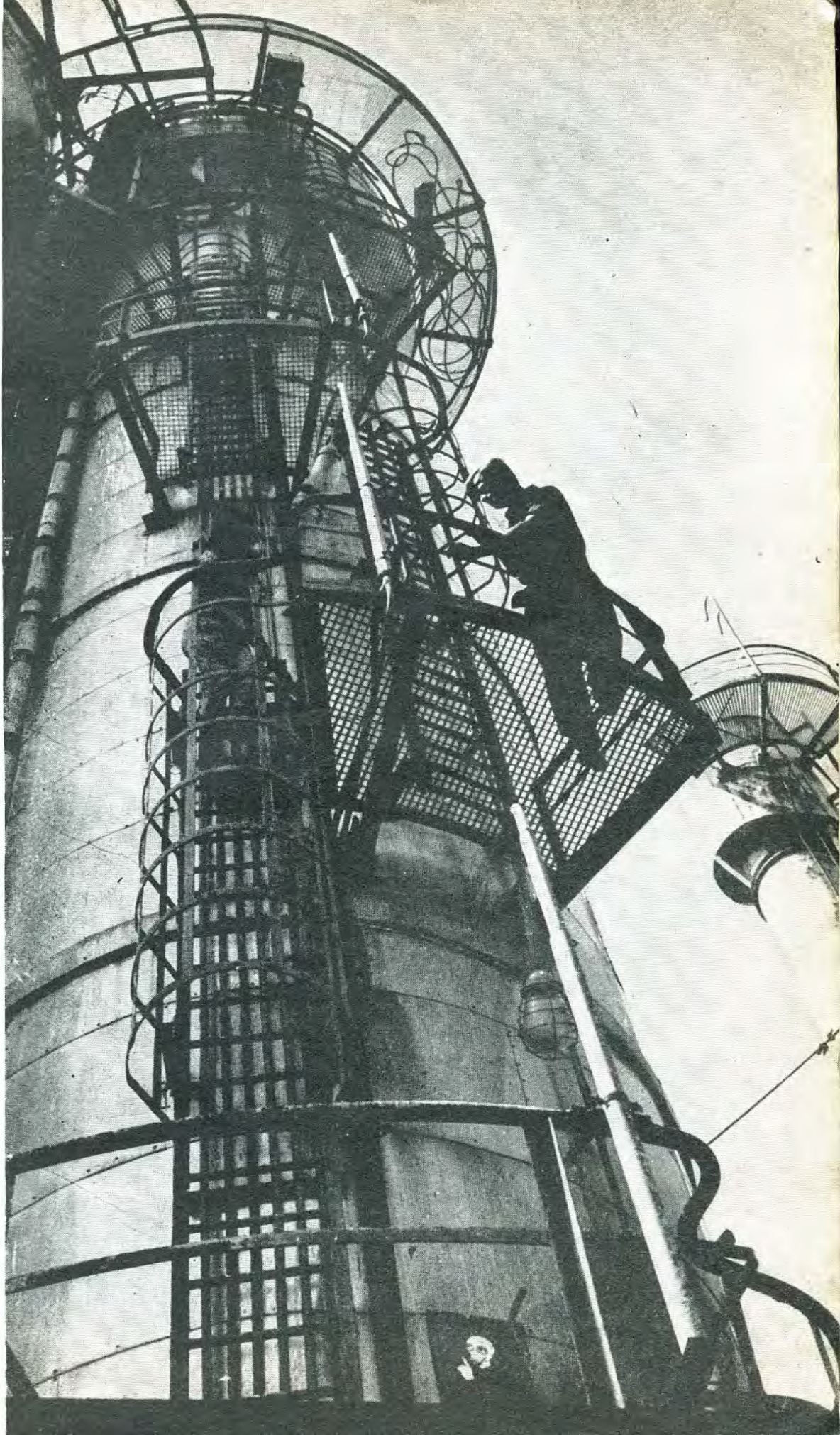
At the Fieri industrial complex
