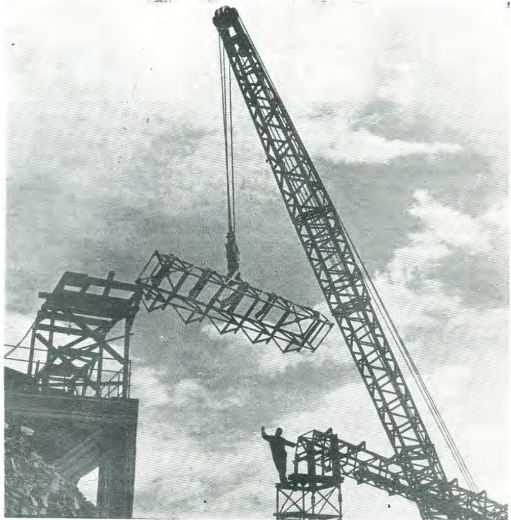
Assembling of new industrial units
